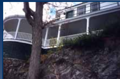
Restoration of facilities for INS in New York State
